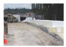
Expanded polystyrene lightweight fill, which is only 1/100th the weight of typical soil, was shaped and placed on the west approach to avoid adding weight above an existing sewer line and minimize settlement of the soft in-situ soils.
