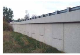
A total of about 18,000 ft<sup>2</sup> of walls were used on both approach fills.
