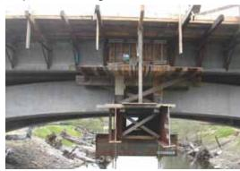
Support for the precast concrete girders was provided at the arched superstructure's apex with a cast-in-place concrete crossbeam.
