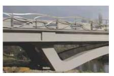
The shape of the substructure arch is flat enough that it functions partially as an arch and partially as a beam. It was cast in one continuous pour to ensure a smooth surface.
