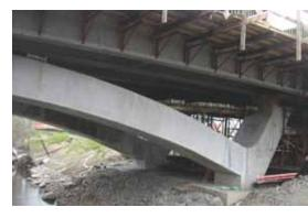
To provide a robust foundation for the columns on both sides, 120-ft-long castin-pipe concrete piles were used to carry both gravity loads and thrust from the arch. At each column pier, a crossbeam was constructed on falsework to support the precast concrete girders and deck.
