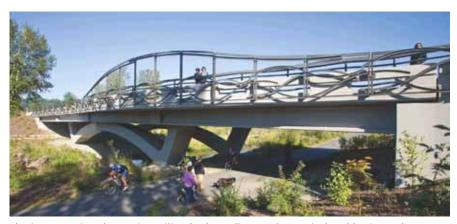
The interweaving decorative railing had to adjust to the vertical and horizontal curves and asymmetrical shape of the bridge, which included sloping bulb-outs on each side to provide lookouts for pedestrians.
