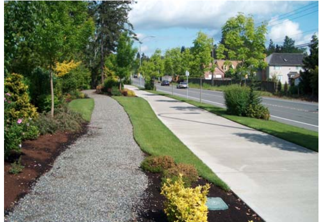
NE 116 th Street in North Redmond features vehicle lanes, bike lanes, a sidewalk, a soft surface trail, and ample greenery.
