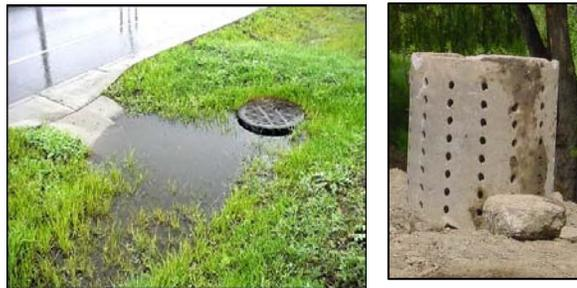
**Typical UIC stormwater wells (drywells)**
