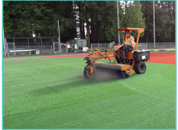
PHOTO: Hartman Park field improvements
