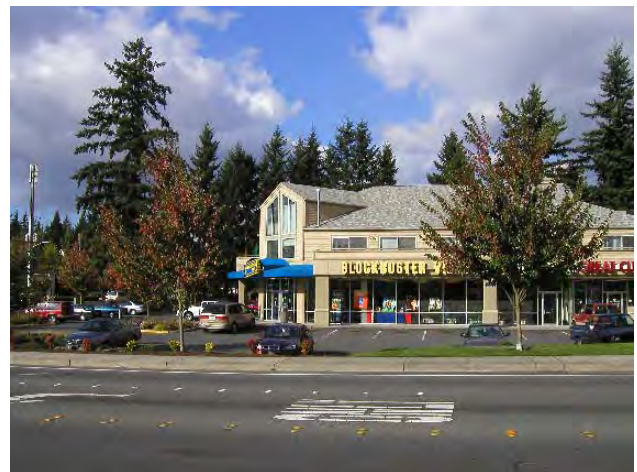
Corner shopping center in the Grass Lawn neighborhood.
